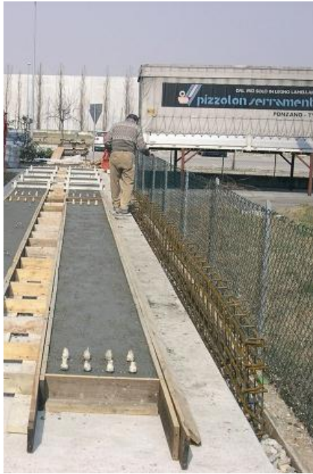
Figure 1 Field tests on restrained drying shrinkage of concrete slabs (8 m long, 400 mm wide and 60 mm thick)
