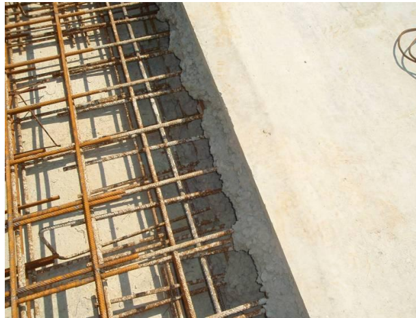
Figure 4 Daily joint crossed by structural reinforcement
