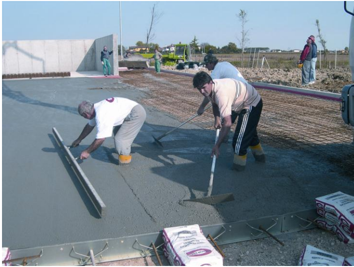
Figure 6 Placing of SRA-PCS-Mix in the concrete floor in the presence of the steel mesh
