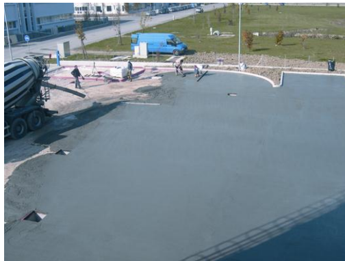
Figure 6 Placing of SRA-PCS-Mix in the concrete floor in the presence of the steel mesh
